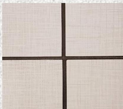
**Using a multi-unit grid keeps grout joints aligned, but the joints' widths vary due to variations in tile size.**
